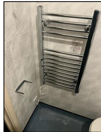
New heated towel rail installed
