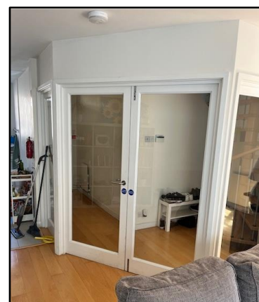
This work physically separated the means of escape thereby improving fire safety
