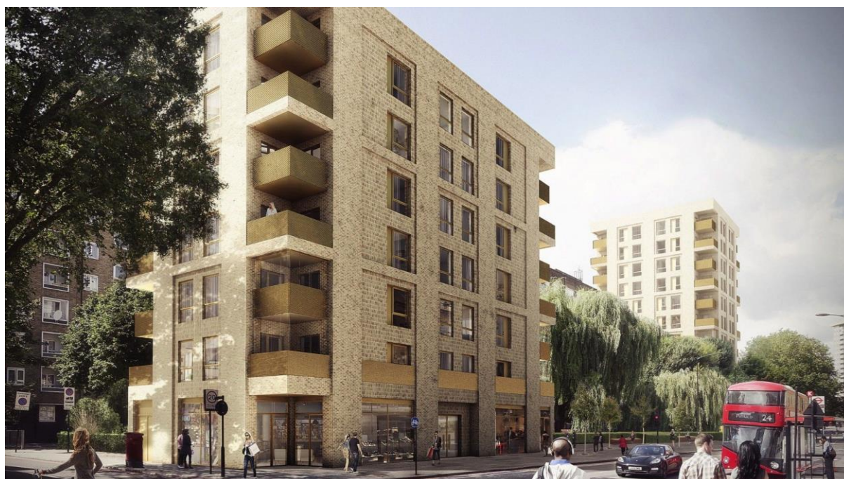
Figure 8. New homes which have recently been provided in the Euston area
